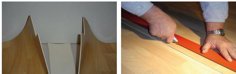
Scrap piece placed under the seam - double cut with a straight edge
